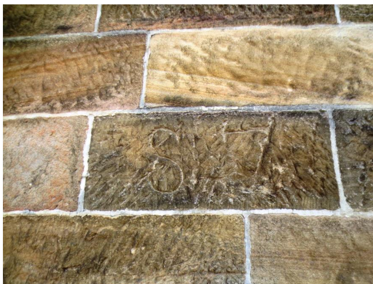
Figure 21 Darlinghurst Gaol wall markings
