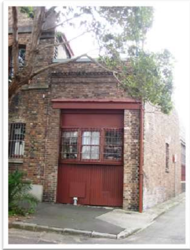
Figure 22: former United Carriage Works (No 42)
